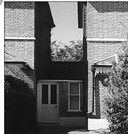
Below right: Adding a first floor to one of two adjoining ground floor annexes would normally be unacceptable.
