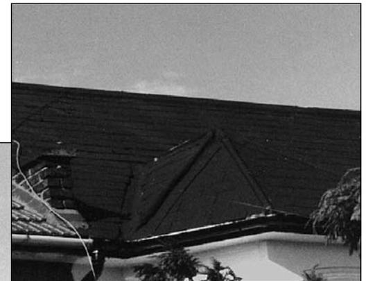
*Concrete tiles and roof sealants as shown here look very different from slates and so must not be used on Woodgrange houses.*
