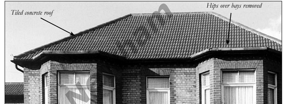
*Altering the original roof shape and materials destroys the character of individual houses and the coherence of terraces.*
